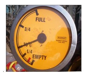
Fig 1 – Magnetic oil level gauge (MOLG)
