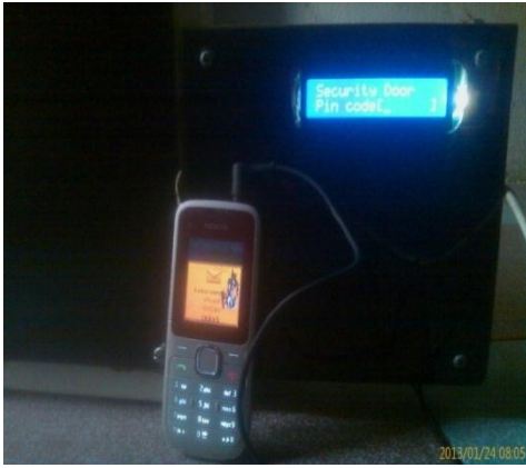
Exterior view of controlling unit
