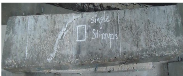
Fig 4.3 Failure of beam H-CB1
