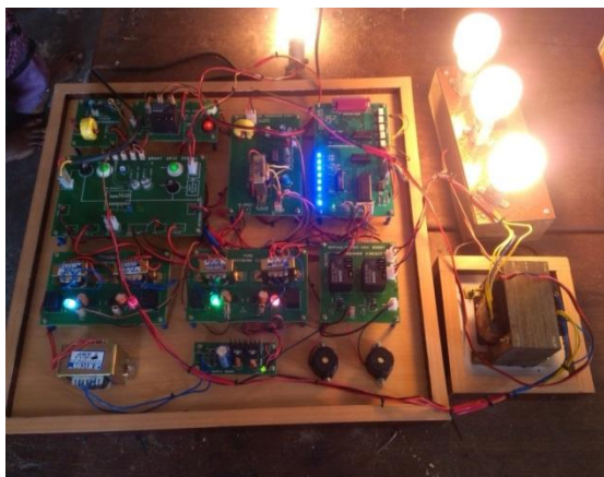
Fig.1 Hardware prototype of fuse monitoring and voltage control
