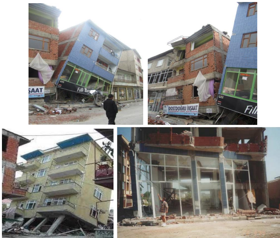
Figure 10 Soft story failures [9-10]
