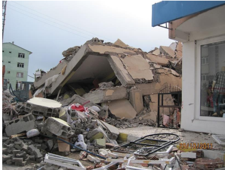
Figure 5 Failure due to column orientation
