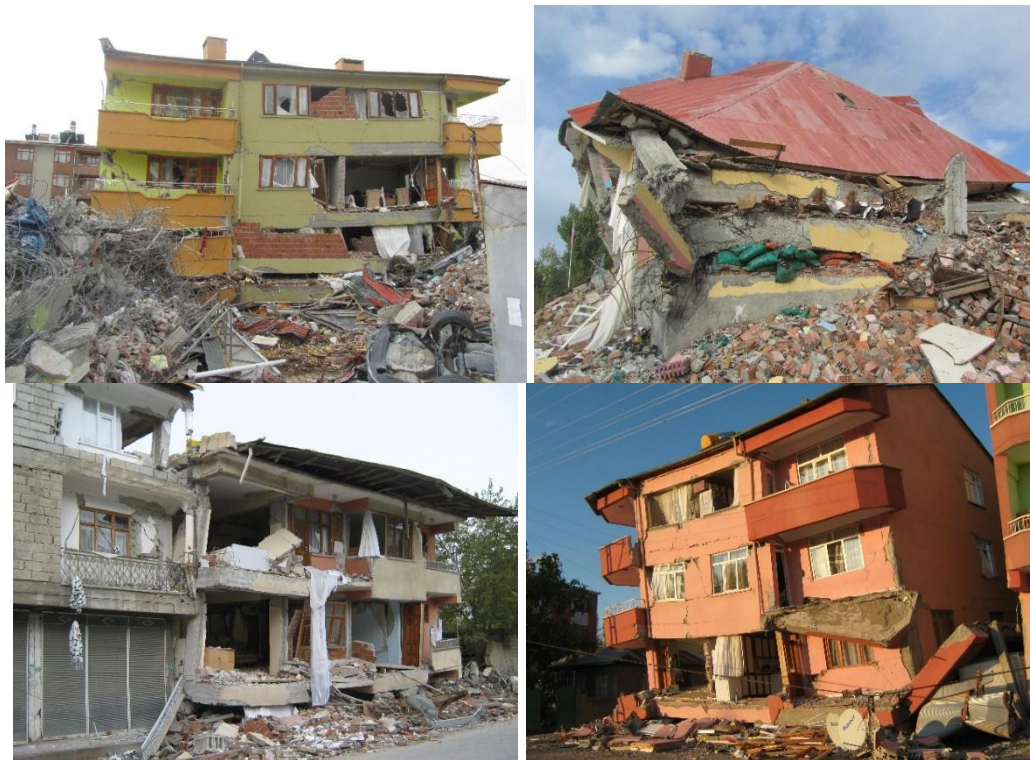
Figure 3 Failure of RC building due to insufficient lateral rigidity
