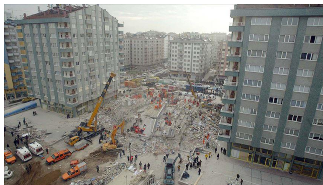
Figure 2 Failure of Zümrüt Apartment [8]
