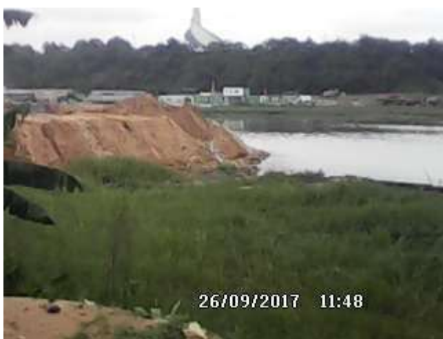
Photo 3: Installation of cement company and backfilling of Banco Bay in Attécoubé
