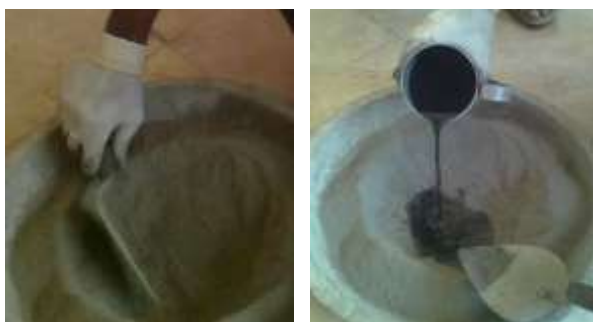
Fig. 5 dry cement, sand and zeolite mixture and adding of MWCNT solution into the dry cement, sand and zeolite mixture
