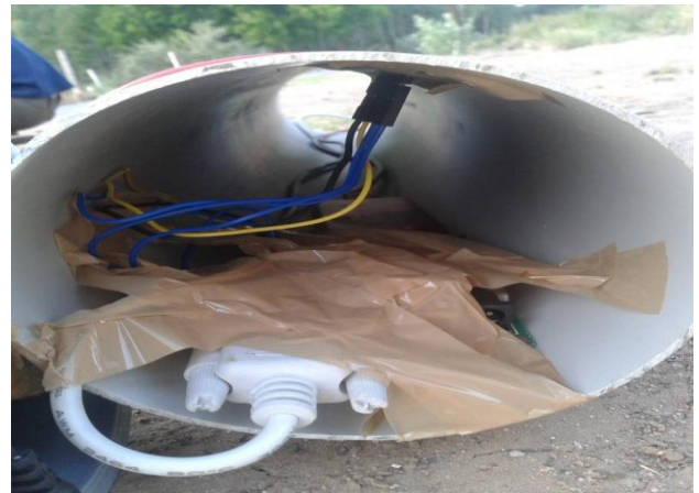
Figure 9: Sensor in pipe
